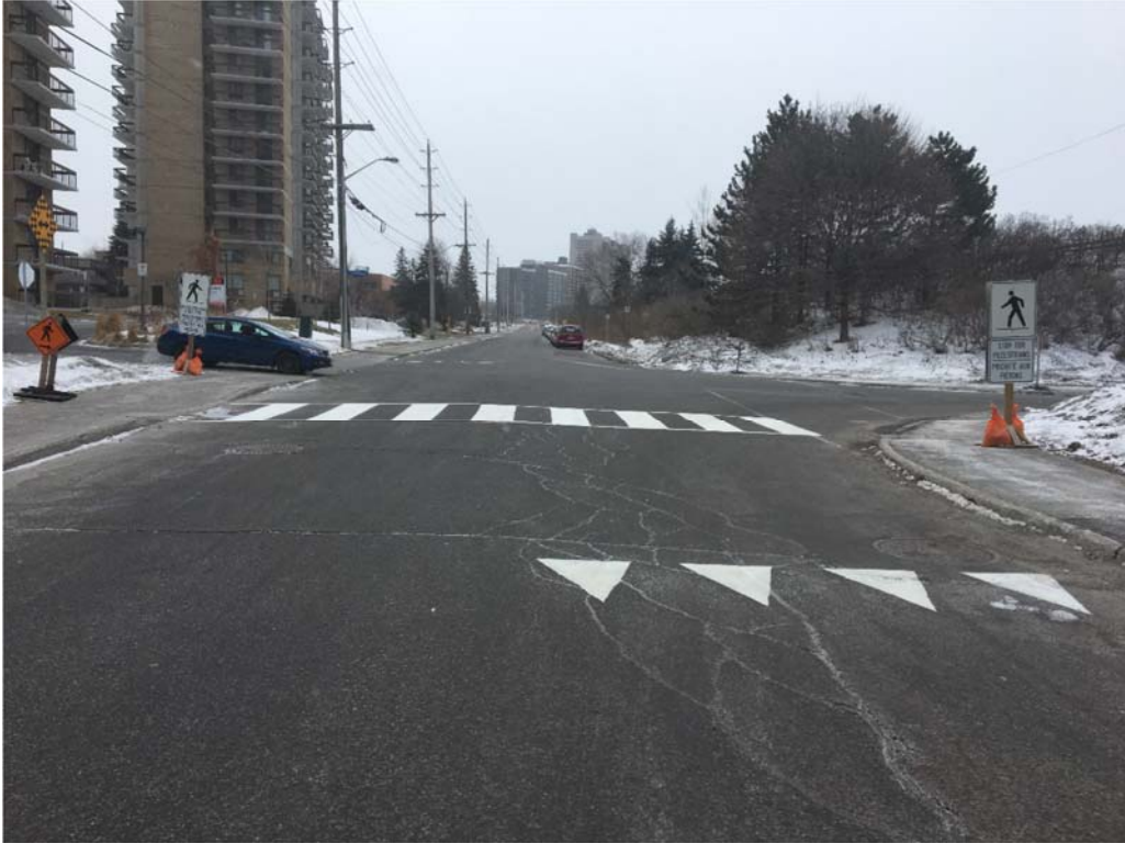
Pedestrian detour signage and line painting (shown looking southbound on Old Riverside Drive at Hincks).
